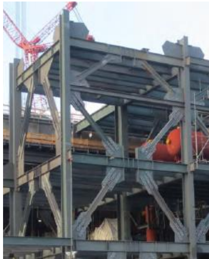
Braced Frame Design
