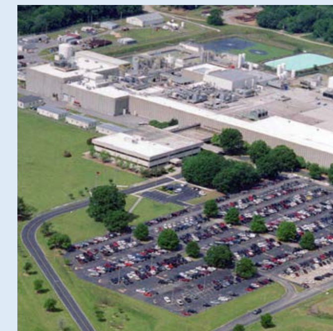
Fuel Fabrication Columbia, SC (USA)
