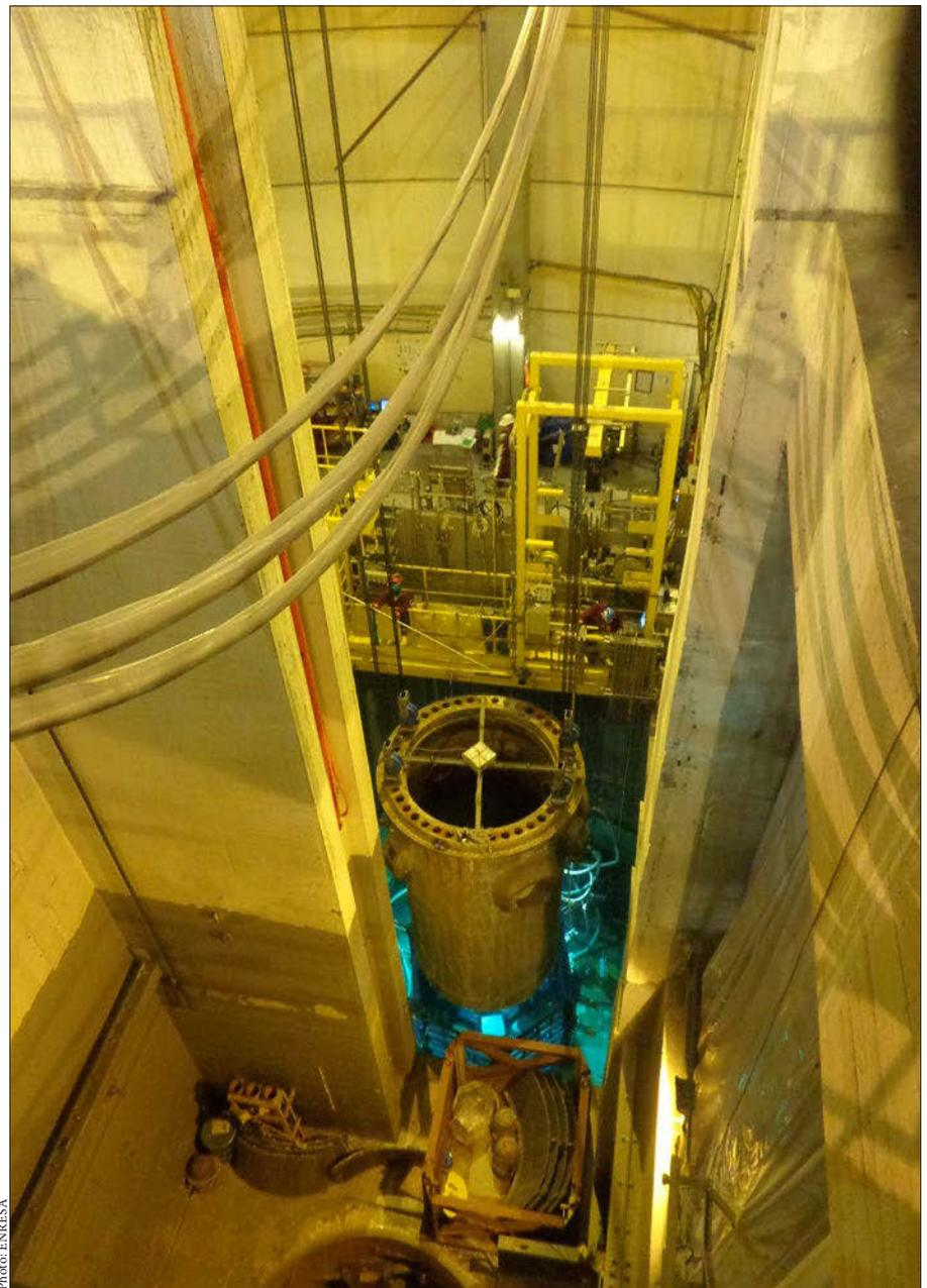
Demolition of the wall separating the reactor cavity and the spent fuel pool at José Cabrera.
