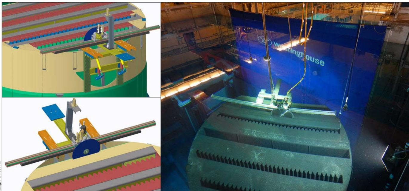
3-D modeling helped determine how to cut the Barsebäck-2 plant steam dryer.
