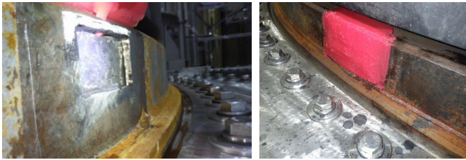
Example of sealing on reactor Vessel flange during outage
