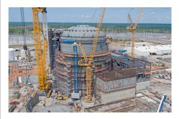
Modularization allows many more construction activities to proceed in parallel and improves quality and efficiency by increasing factory-based manufacturing and assembly.
