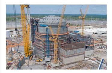
Modularization allows many more construction activities to proceed in parallel and improves quality and efficiency by increasing factory-based manufacturing and assembly.
