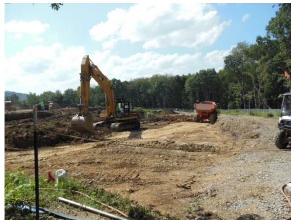
Site Remediation: Screening
