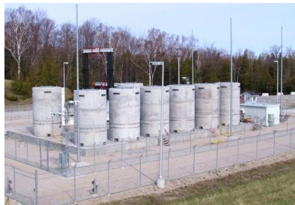
Typical Independent Spent Fuel Storage Installation.
